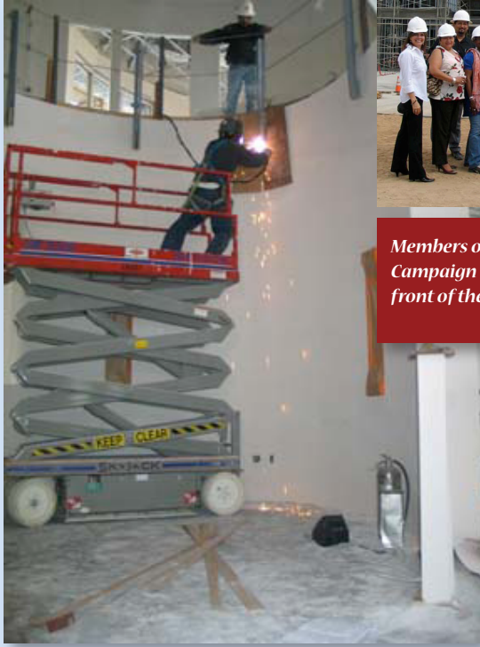
Sparks fly in the first floor reception area of La Maestra's new health center.
