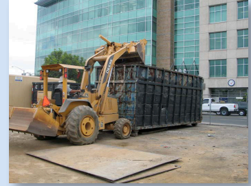
La Maestra's "green" construction team has followed an aggressive recycling program throughout the project.
