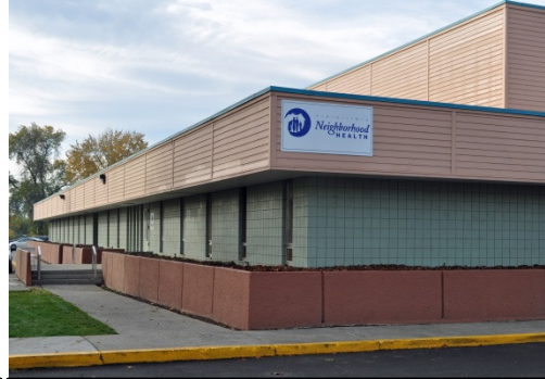
Southeast Community Center
