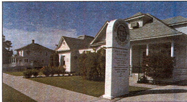
Today, the Yakima campus of Neighborhood Health Services extends over much of a full city block in downtown Yakima. The collection of early Yakima homes has been connected, lovingly restored and thoroughly modernized – transformed into contemporary medical and dental offices, exam rooms, offices and meeting rooms. "We are committed to neighborhood improvement and retaining the character of the community," says Chief Executive Officer Anita Monoian. "These houses have become a symbol of our past and future. They capture the spirit of the place."
